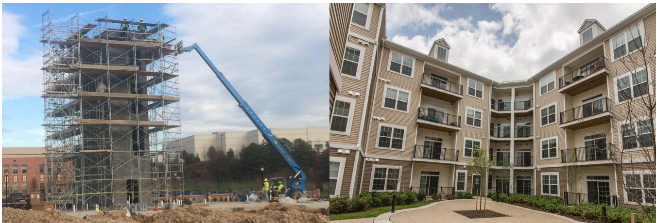
Oxford Square construction.
