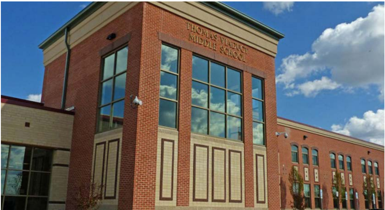
Thomas Viaduct MS opened in August of 2014
