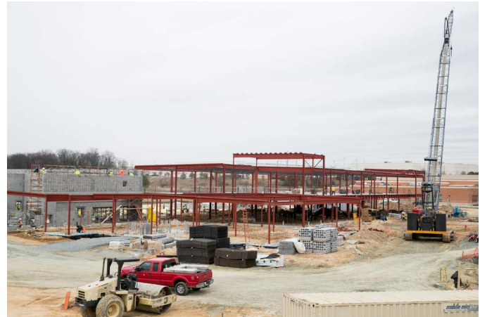
Construction of New ES #42.
